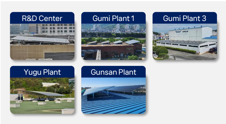
| Solar Power Generation Sites
